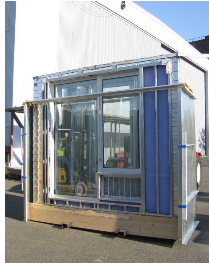
OFF-SITE ELEMENT READY FOR INSTALLATION
